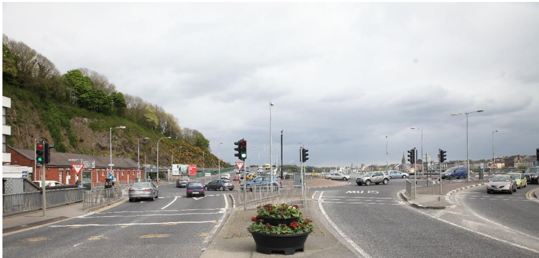
Plate 1.2 Traffic on the Plunkett Station roundabout, looking east showing the absence of cycle lanes
